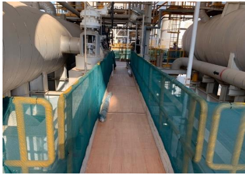
Material fall protection on Walkways and hand rails
