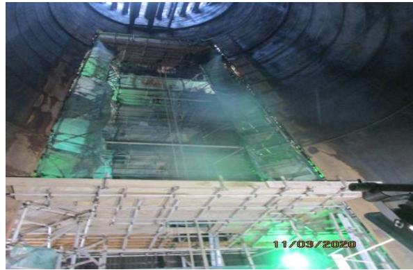
Safety net provided on external and internal scaffolds.
