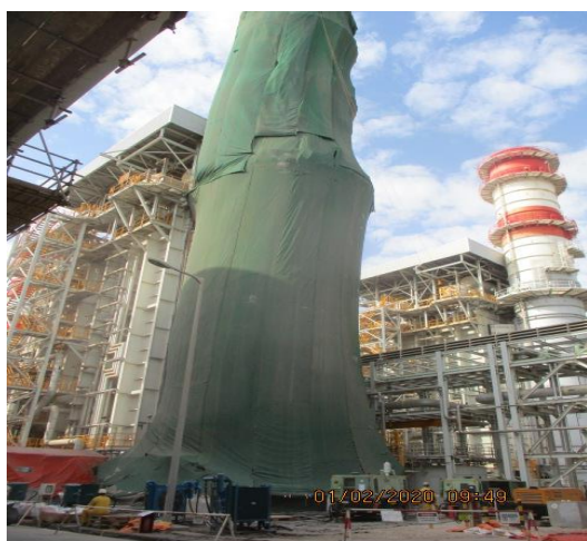
Main Stack Painting and Sand Blasting Activities – Stack fully covered
