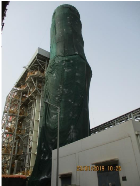
Main Stack Painting and Sand Blasting Activities – Stack fully covered
