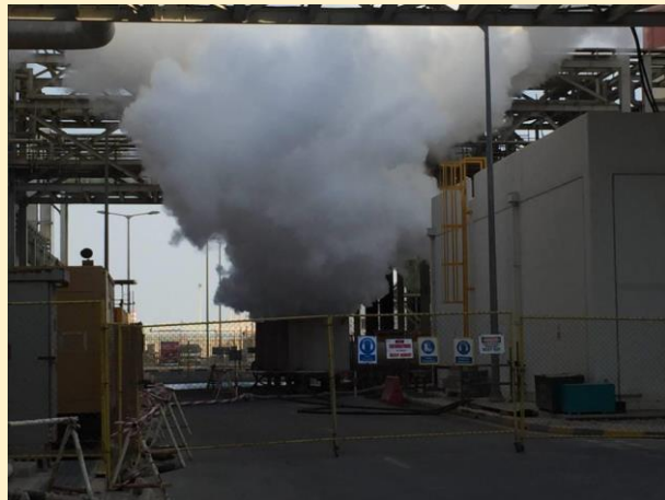
Steam blowing area controlled with fencing, sign boards and monitoring noise level
