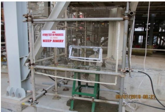
Hydro Test Area – Monitoring Gauges area protected using wire net.
