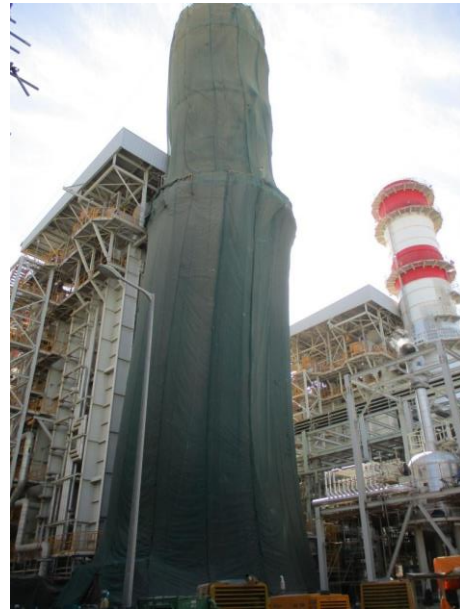
Main Stack Painting and Sand Blasting Activities – Stack fully covered
