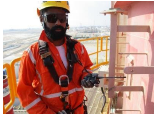
Rope access painter with complete PPE's and walkie talkies
