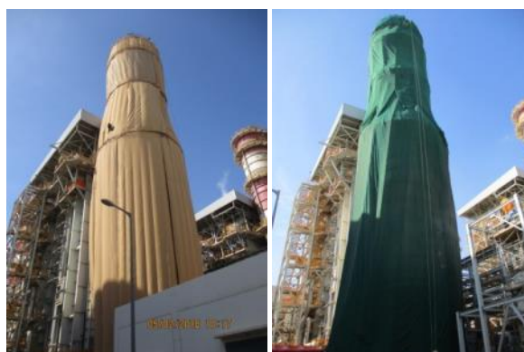
Main Stack Painting and Sand Blasting Activities – Stack fully covered
