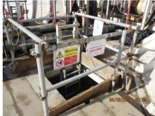
Confined space access with barricade and signage's
