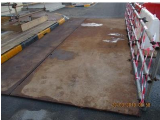
Steel ramp and hard barricades in excavated area
