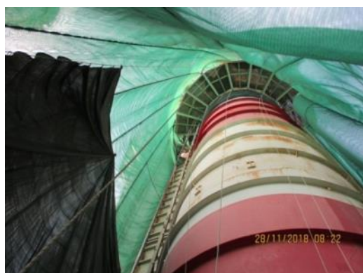
Main Stack Painting and Sand Blasting Activities – Stack fully covered
