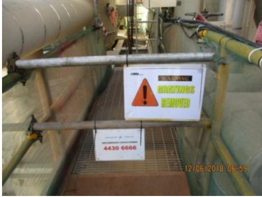
Floor grating removed areas are hard barricaded
