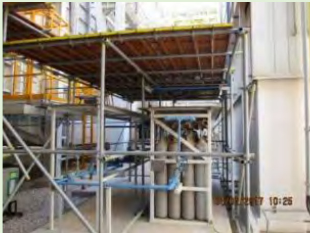
Compressed Gas Cylinder Storage Area Protection
