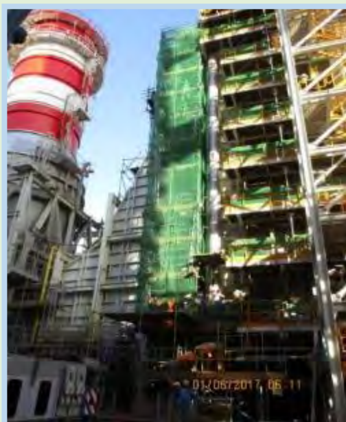
Safety nets provided on scaffold tower
